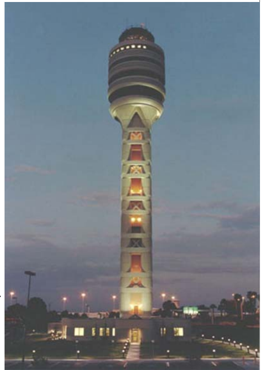
Air Traffic Control Tower Orlando Florida
